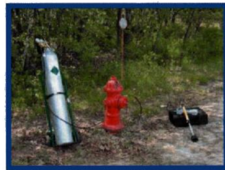
Leak Locating on City Water System
