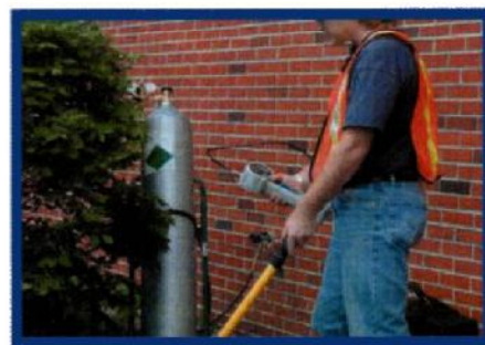
Leak Locating on Residential Supply
